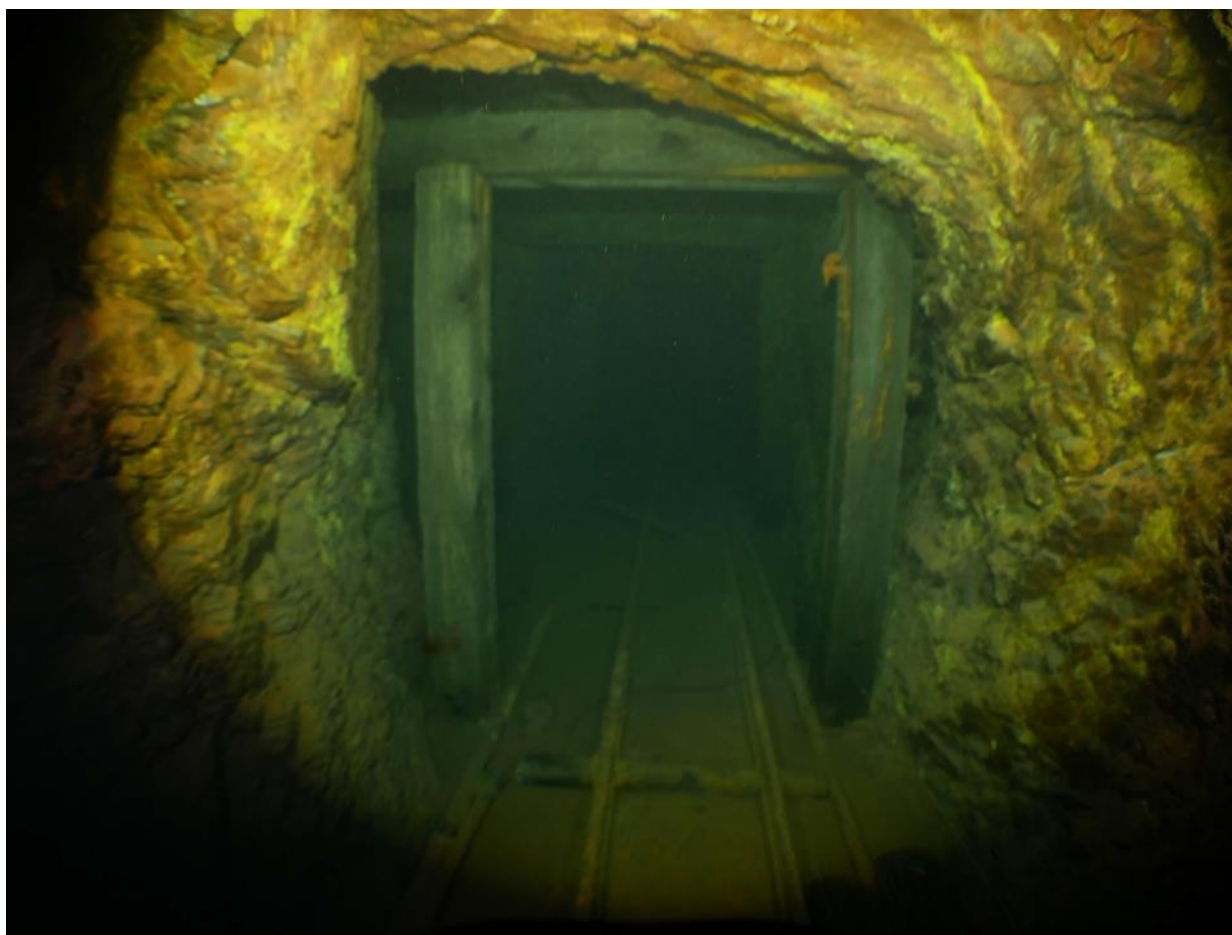
Figure 84. Image of the mine's drift supported by beams. The small gauge rail can be seen running along the floor and a candle holder is still attached to the right wooden beam. (Leah Potts)
