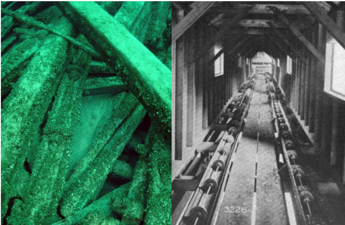
Figure 43. Transfer 's longitudinal, Cable Conveyer and the Jeffery Manufacturing Co. Cable Conveyer (Wisconsin Historical Society, Jeffery Manufacturing Co.)
