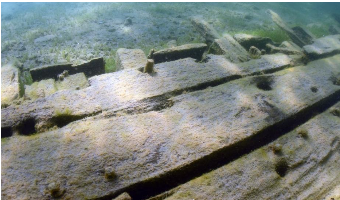
Figure 7. Ceiling planking, frames, and covering board (Wisconsin Historical Society)
