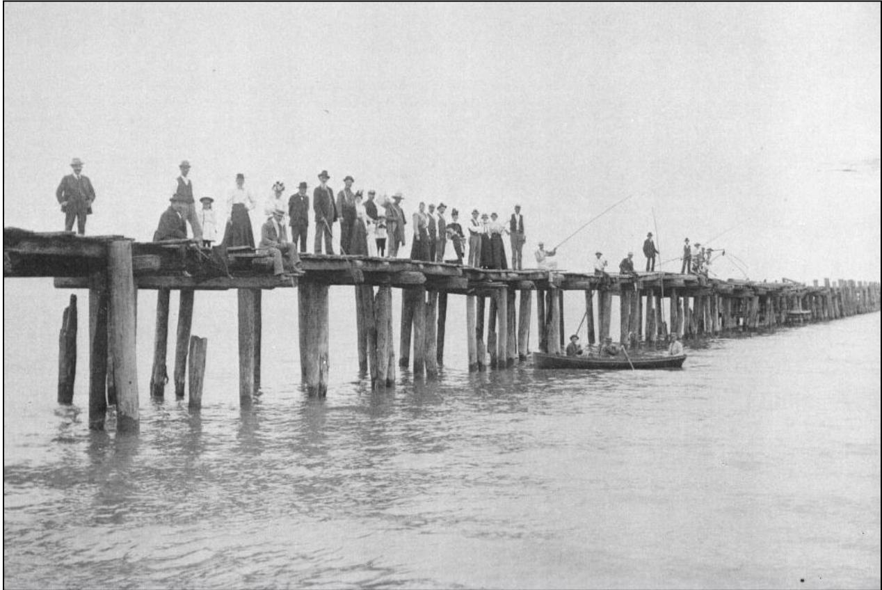
Figure 10: One of the twin piers at Centerville (also called Hika, and now within the municipal boundaries of Cleveland, Wisconsin), ca 1895-1910 (adapted from Village of Cleveland 2020). Note evidence of repair/rebuilding in the form of older pilings.
