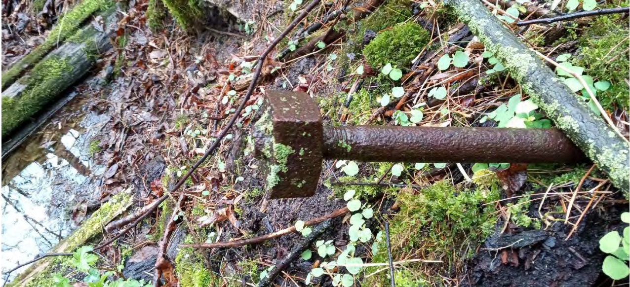
Figure 69: Tie rod extending outward from corner of pit within structural feature. An identical rod lies on the ground surface on the opposite corner of the pit.
