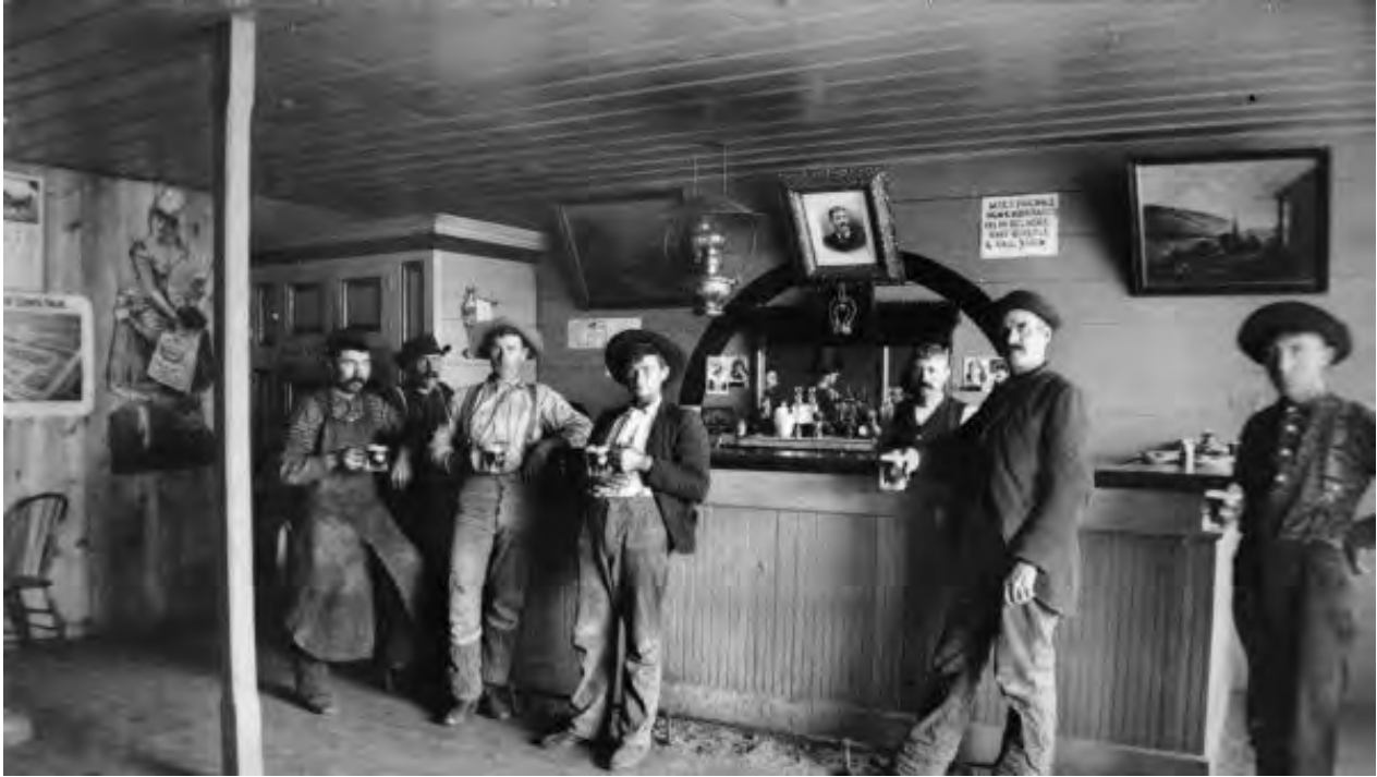
Figure 127: Workmen in a northern Wisconsin saloon, ca. 1892. Wisconsin Historic Image 55795.
