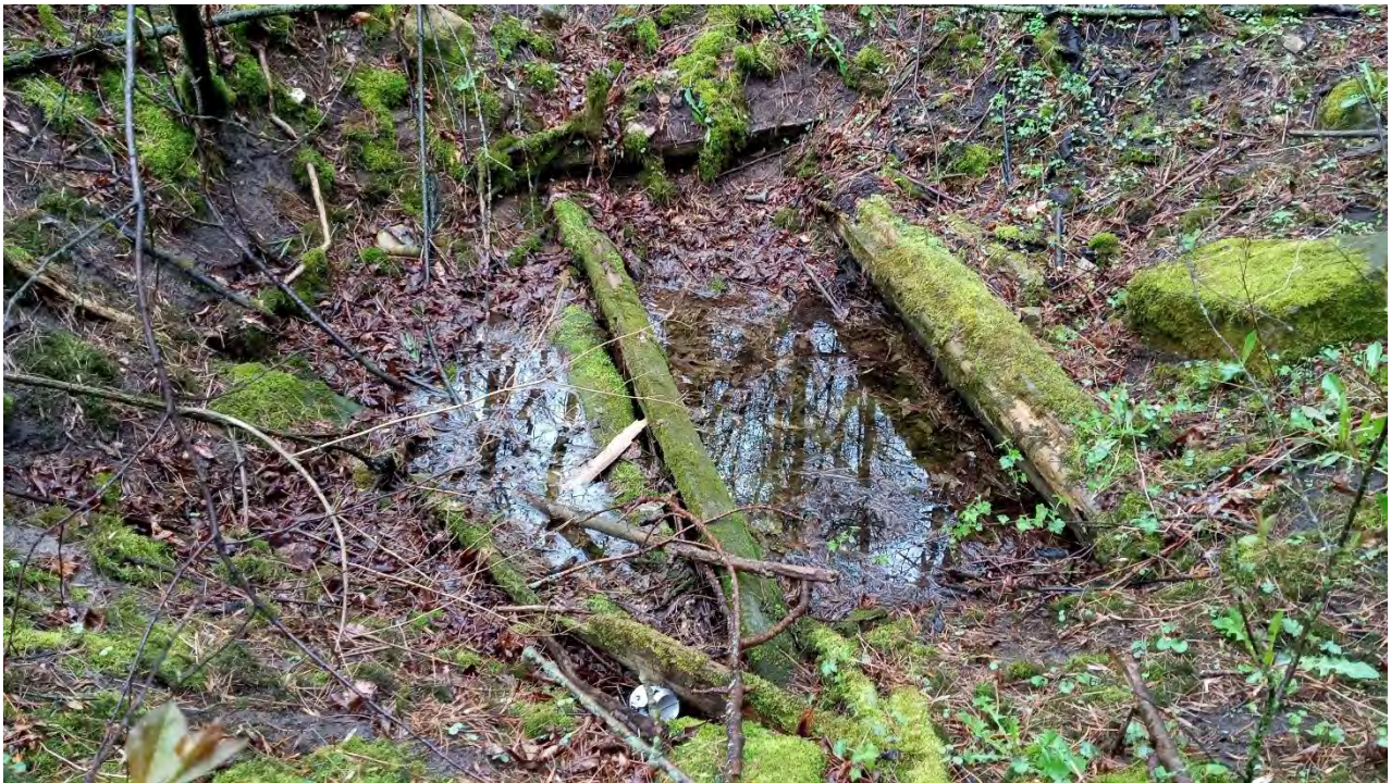
Figure 68: Pit within structural feature. Note timber and plank framing within pit.
