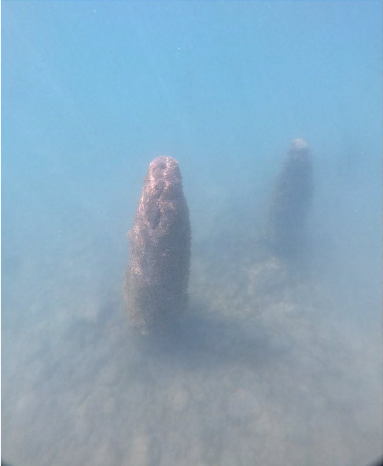
Figure 110: Submerged pilings at Alaska pier, 2022.
