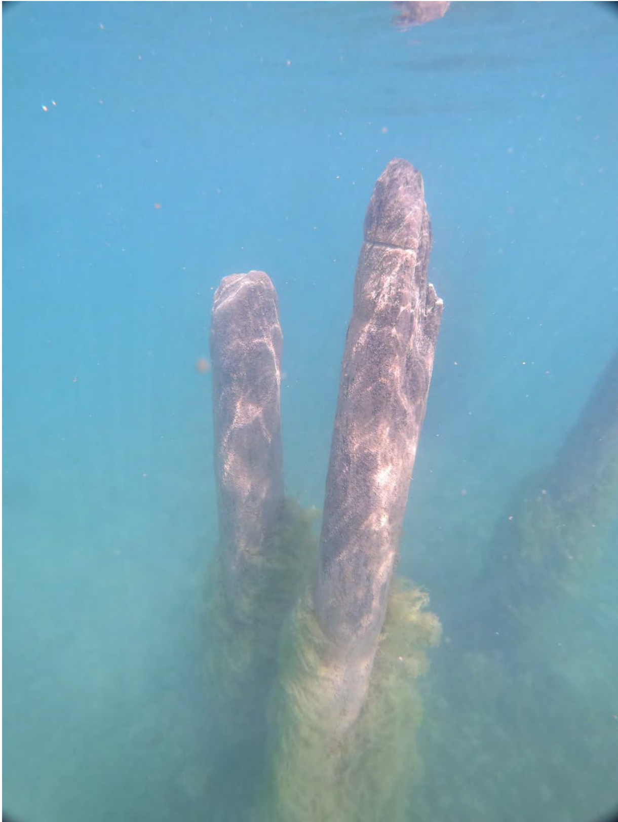
Figure 61: Pilings belonging to Dean's pier. Photo taken 2022.
