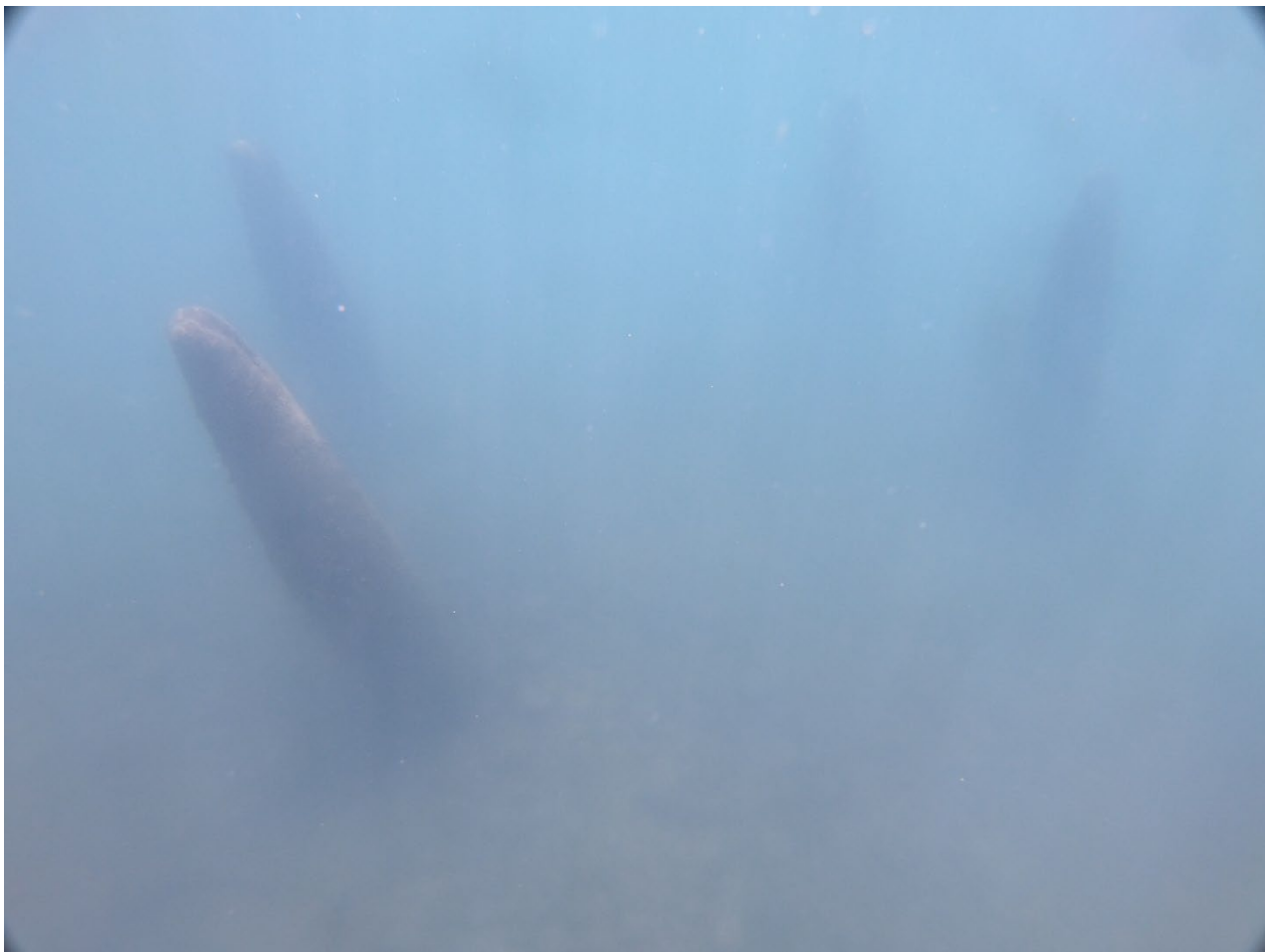
Figure 111: A cluster of pilings at Alaska pier, 2022.
