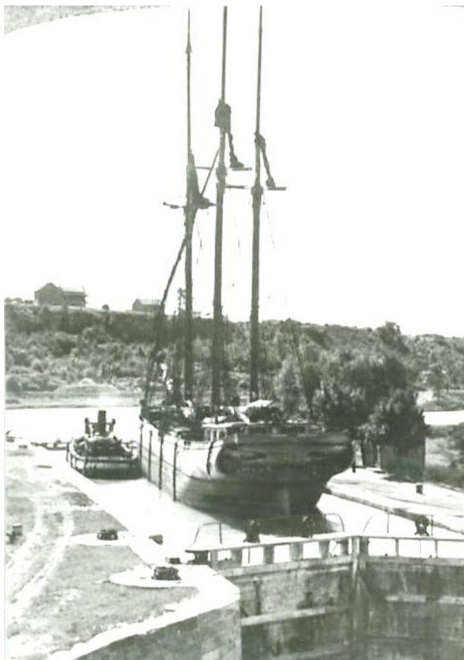
Figure 7. Sailing canaller Arthur in the Welland Canal locks near Thorold, Ontario. After the third expansion in the late 1880s, the locks were wide enough for tugs to escort vessels within the locks and through the canal. (Public Archive of Ontario)
